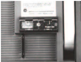
Limited access pushbutton cover
