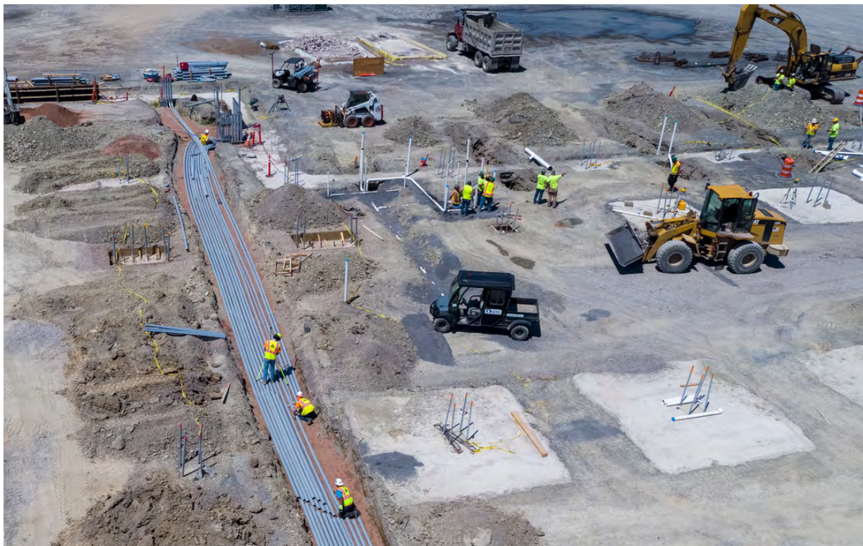
This aerial view shows electricians working in the field using a digital system to lay out conduit. Photo courtesy of O'Connell Electric
