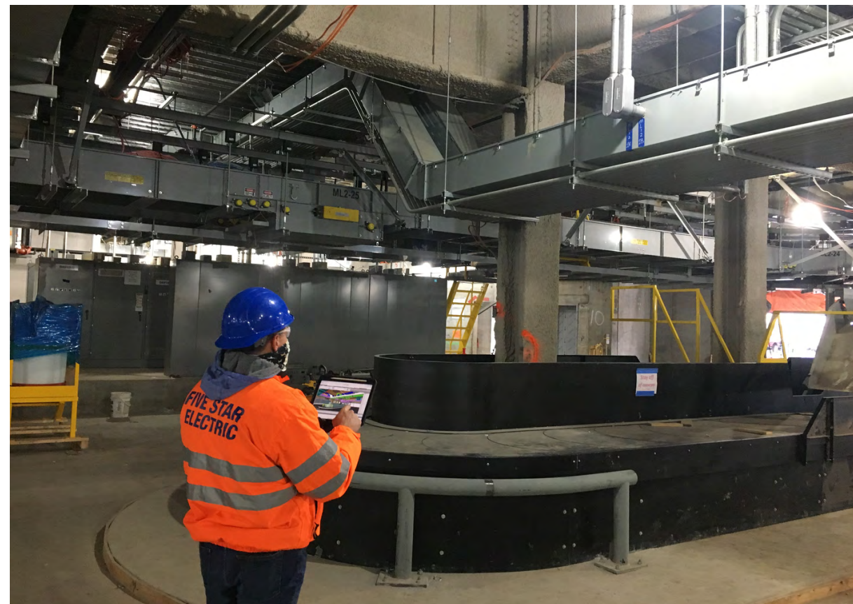
A Five Star Electric project manager compares the BIM model to physical installation at the Newark Airport Terminal One project. Photo by Brian Leonard, courtesy of Five Star Electric
