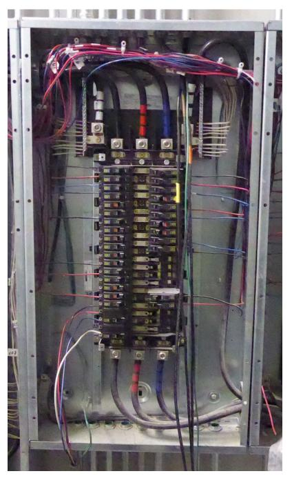
**Photo 1.** Phase conductors terminate down into the panel's main lugs. As outlined in the new version of IEEE 1584, this would be best modeled as a VCBB conductor configuration.
