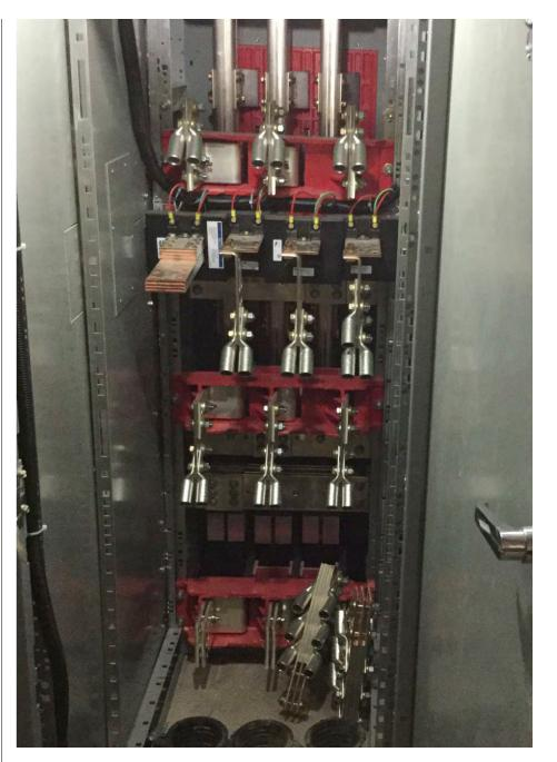
**Photo 2**. These draw-out circuit breaker compartments (as seen from the rear of a switchgear cabinet under construction) house connections that run horizontally from the circuit breaker stabs to the switchgear bus. Within the breaker cell, an operator would be exposed to conductors in the HCB configuration.
