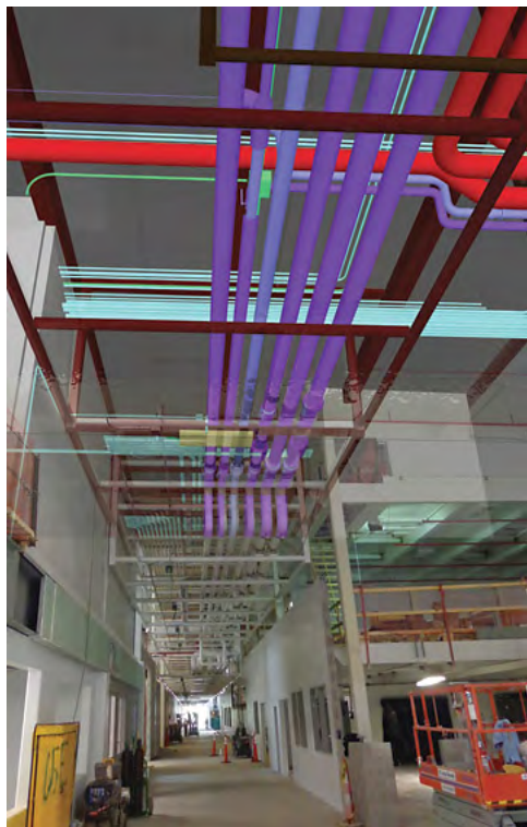
This image shows the alignment of the model and the real-world conditions for a pipe and electrical rack for a project in Topeka, Kan.
