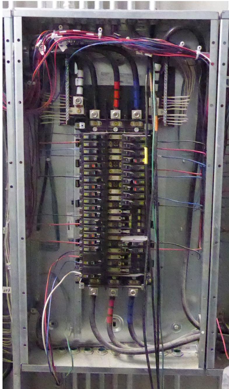
**Photo 1.** Phase conductors terminate down into the panel's main lugs. As outlined in the new version of IEEE 1584, this would be best modeled as a VCBB conductor configuration.
