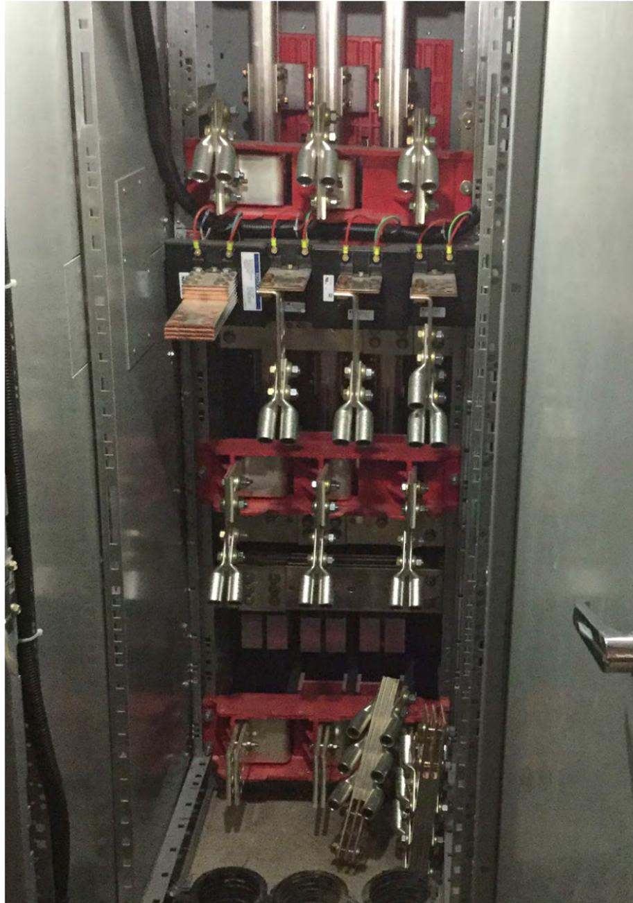
**Photo 2.** These draw-out circuit breaker compartments (as seen from the rear of a switchgear cabinet under construction) house connections that run horizontally from the circuit breaker stabs to the switchgear bus. Within the breaker cell, an operator would be exposed to conductors in the HCB configuration.
